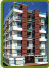
Geo Tomal-Tanuka House :14, Road No : 12 Sector No : 13, Uttara, Dhaka Size : 1500 sft
